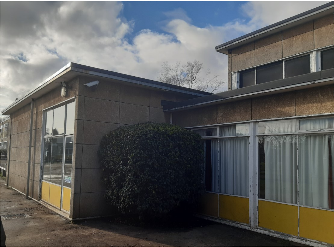
Close up of western range to southern courtyard that shows the original metal glazed screen/fenestration elements and original metal framed windows of the clerestorey to the hall/gym.
